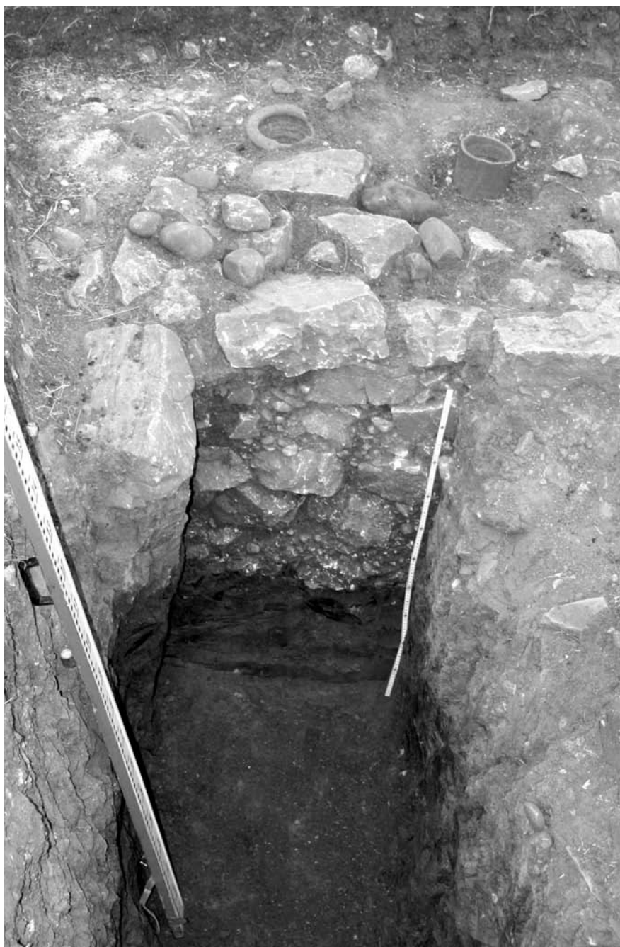
Eastern part of the foundation wall of the structure with embedded ceramic tubuli
