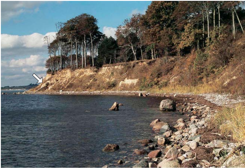
Fig. 42. The Klintinghoved cliff, viewed from the east (cliff is c. 10 m high). The location of the type section of the Klintinghoved Formation is arrowed.
