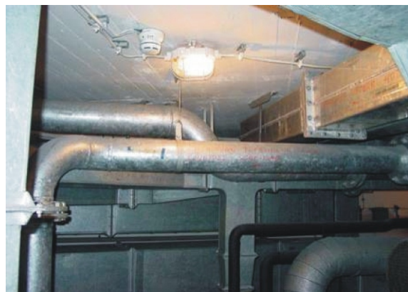
Figure 2. Dismantling metal conducts of the ventilation system
