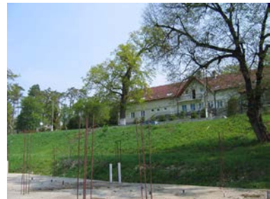
Fig. 7. Rodbav Spa complex, in 2012
