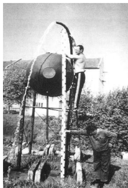
Figure 10 Storage tank at about 4m above irrigation ground level with a leveling staff
