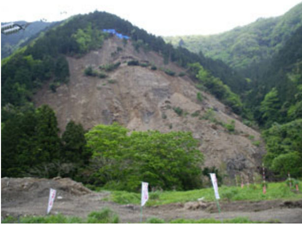
Fig. 5. General view of the landslide site (14 May 2006).
