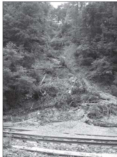
Figure 12. Earthflow from July 2005 Upstream from Lainici Station, which caused the interruption of railway's traffic
