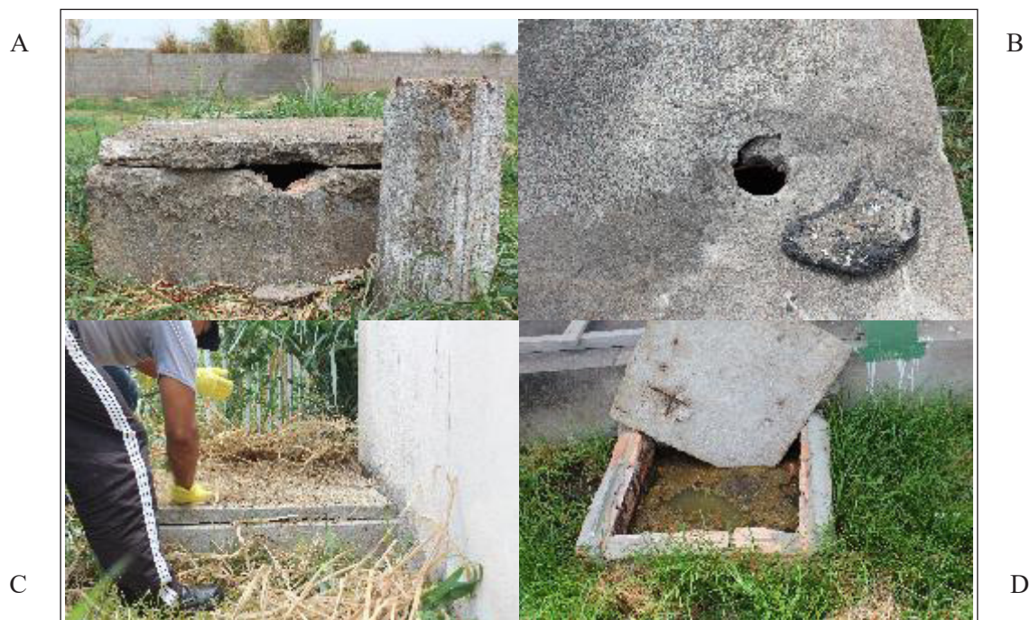
Figure 2 – Points of effluent collection at the General Hospital of Roraima - GHR
