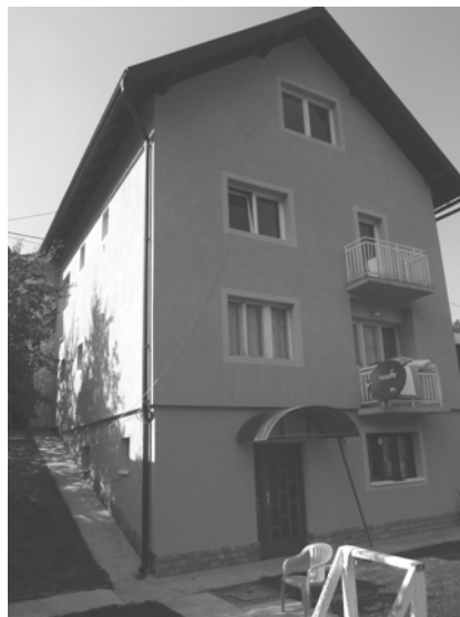
Figure 1. Representative of some of the predominant individual housing unit types in West Serbia region (statistically), a free standing house built in the 1970s
