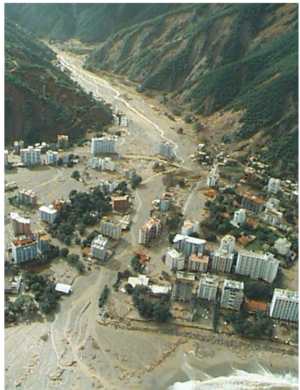
Fig. 2. Communities affected by debris flows and flash floods, Vargas state, Venezuela. A. Cluster of small houses on river flood plain at base of steep hillslope. Note debris-flow scars on hillslopes behind houses. B. Large apartment buildings on alluvial fan at mouth of a river draining the steep mountains of the Venezuelan north coast (Larsen and Wieczorek, 2006).
