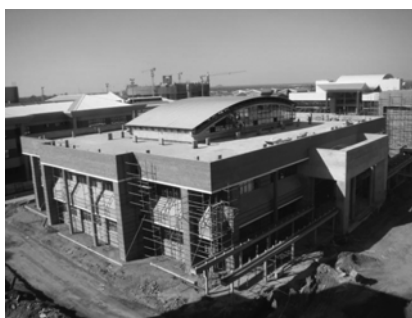
Fig. 4 The new DAP Building, Source: Author's photo, 2011
