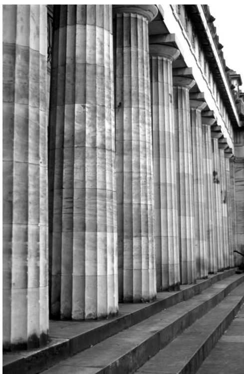
Fig. 3. The requirement for thick continuous beds of good quality sandstone is exemplified by the columns of the Royal Scottish Academy in the New Town of the City of Edinburgh (1826). Stone from Craigleith and other Scottish quarries in central Scotland was used for construction of the columns and for pavement (Photo: A. A. McMillan).
