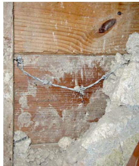
Fig. 9. Barbed wire used as reinforcement for masonry (6)
