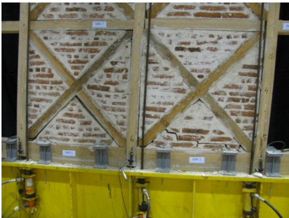
Fig. 8. Separation of masonry from timber frame when subjected to shear stress
