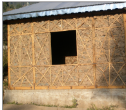
Fig. 4. Housing reconstruction in earthquake affected areas in Pakistan (9)
