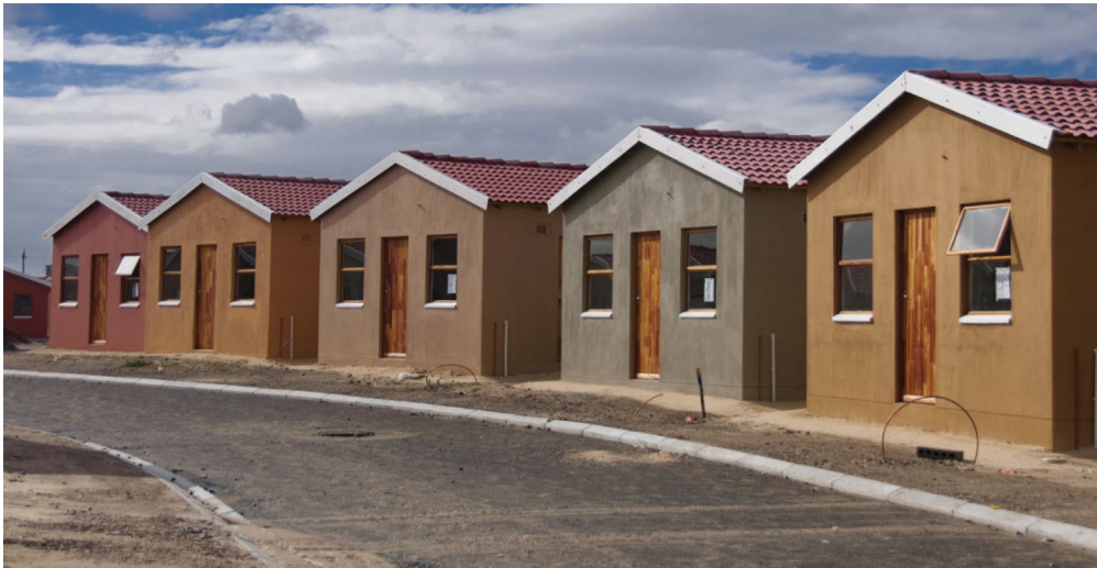
Figure 1.1: Boystown social housing, Cape Town (HDA, 2015)
