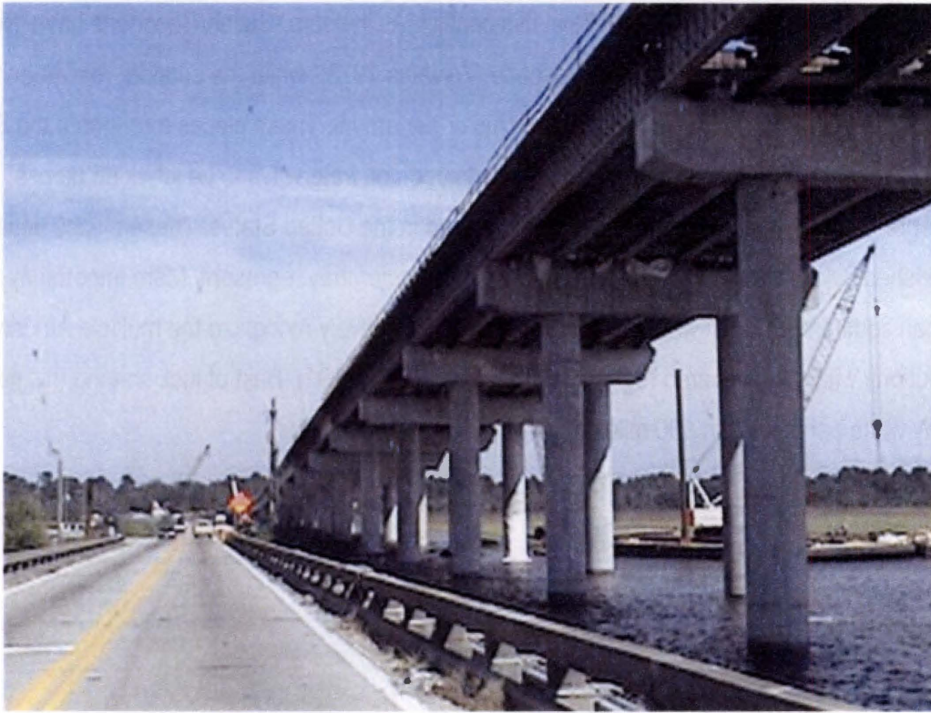
Figure 3.1: An Image of Change (Bridge Construction on Highway 278, Beaufort Co. SC)
