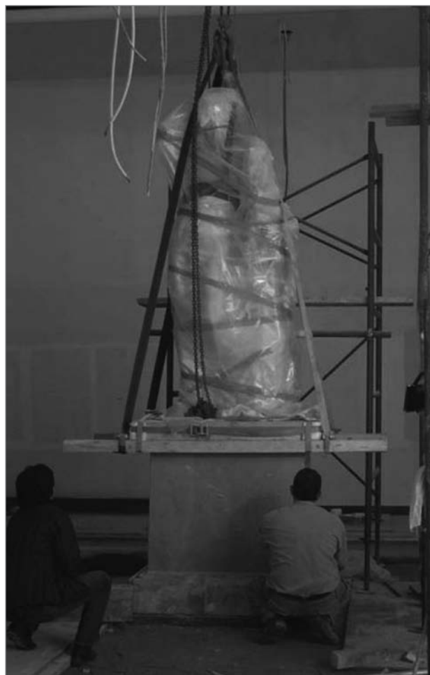
Figure 3: Placing the statue onto seismic isolation (source: Koumouisis, 2007).
