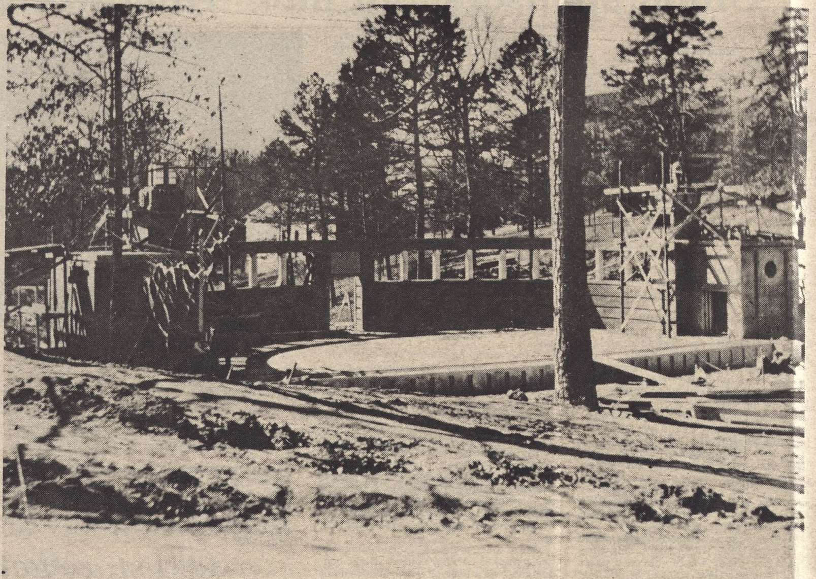
THE CONSTRUCTION OF the outdoor theater began in December 1939. The theater was finished six months later
