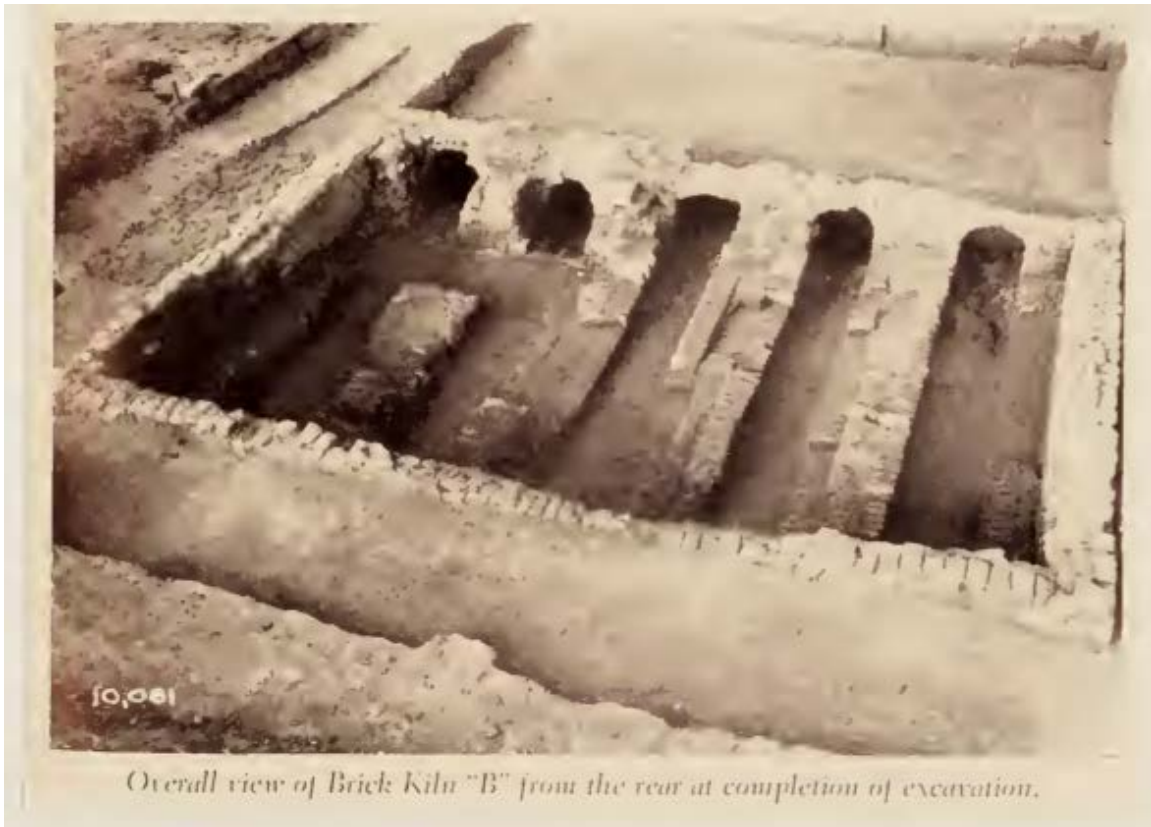
Figure 4.10: Clamp, Below Ground Example. Jamestown, Virginia (Lucy B. Wayne, Burning Brick , 89).
