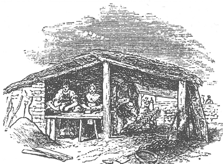
Figure 4.8: Molding Shed (Gerard Lynch. Brickwork: History, Technology and Practice: v.1&2 . (London: Routledge, 2013) 18).
