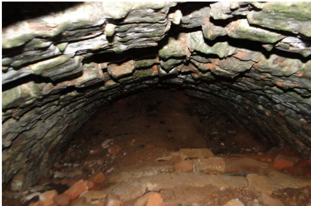
Figure 5.9: Clamp B Passage Interior (Photo Frances Pinto).
