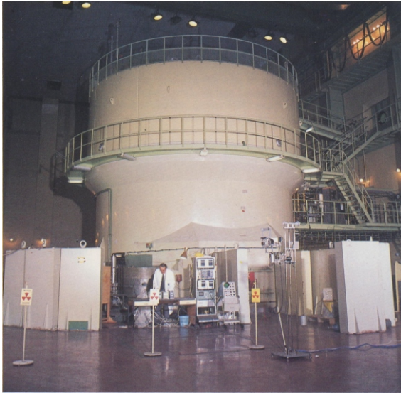
Figure 1. RA research reactor
