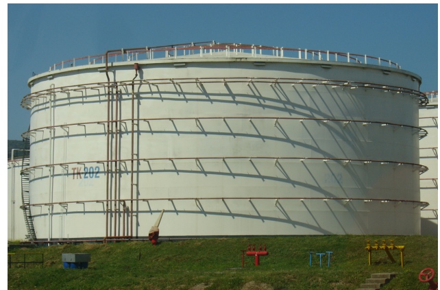
Fig. 3. Retrofitting on the naphtha tank TK-202 burned during the fire.
