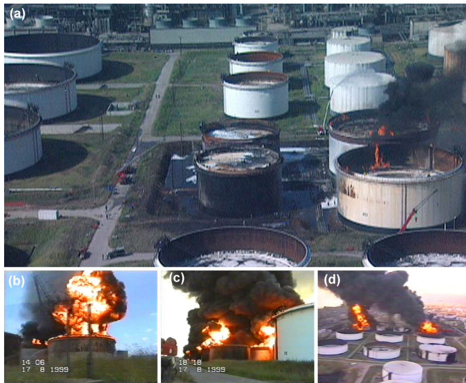
Fig. 1. The progress of the tank farm fire after the flange failure.
