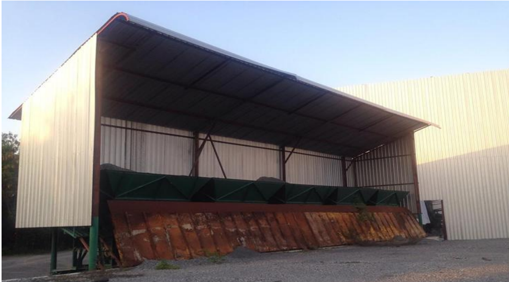
Figure 5: Improvement Shed for Storage Rock Constructed from Metal Sheet
