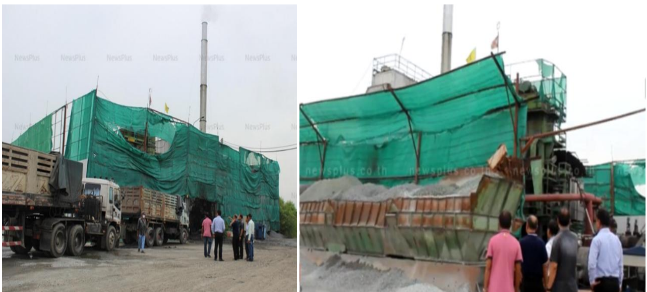
Figure 4: Current Shed for Storage Rock Constructed from Net or Fabric Sieve
