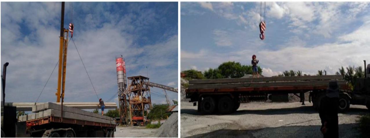
Figure 9: Improved Construction Area Using 5S Practice
