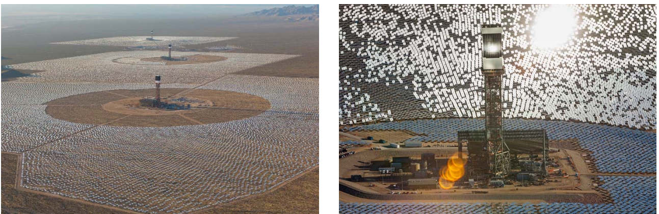
Figure-10: Ivanpah Solar Electric Generating System – (DAILYTECH MAGAZINE, 2017)
