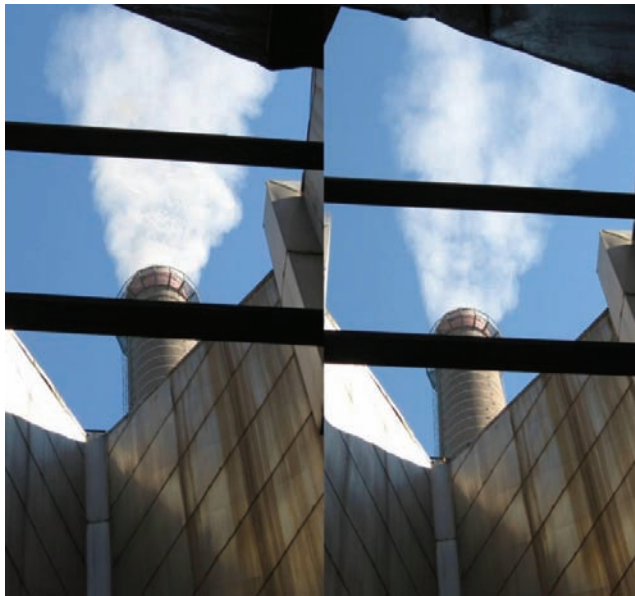
Fig. 14 – The left part of the figure illustrates the smoke appearance in configuration of 4 \times 50\text{Hz} . The right part of the figure illustrates the smoke appearance in configuration of 2 \times 50\text{Hz} + 2 \times \text{HF} .
