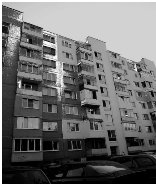
Fig. 8. Block 45, entrances 2-5, Mladost 14
