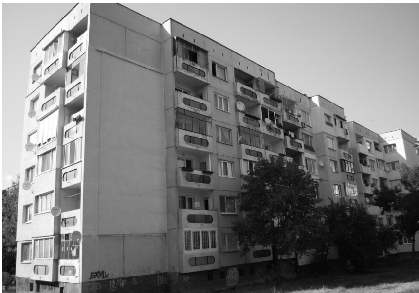
Fig. 5. Side view of Block n. 52, ent. 3, Mladost 1
