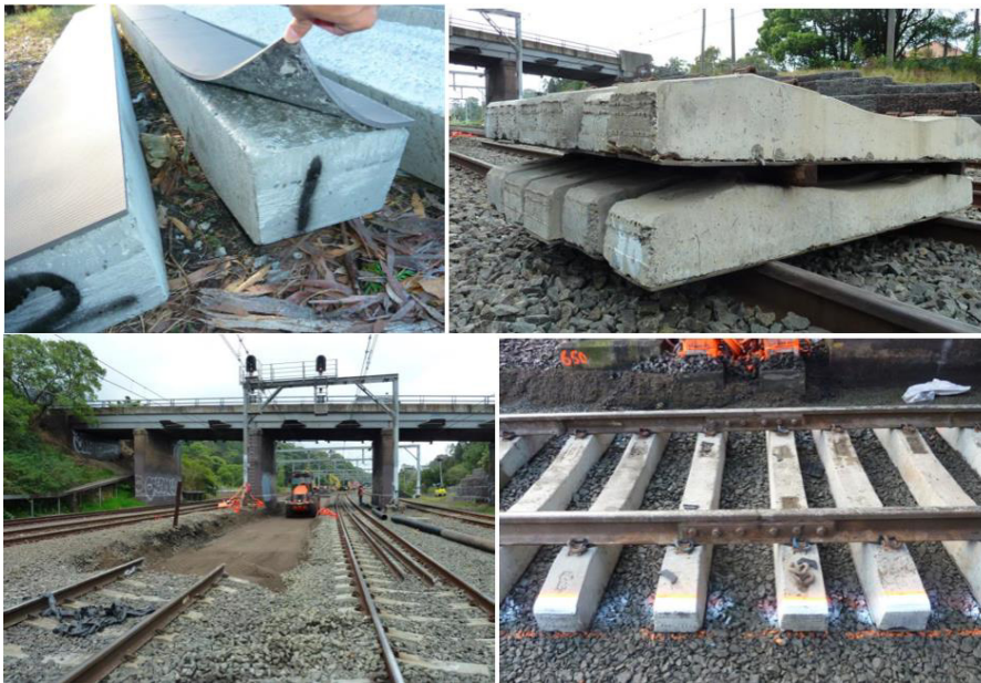
Fig. 3. Field test installation.
