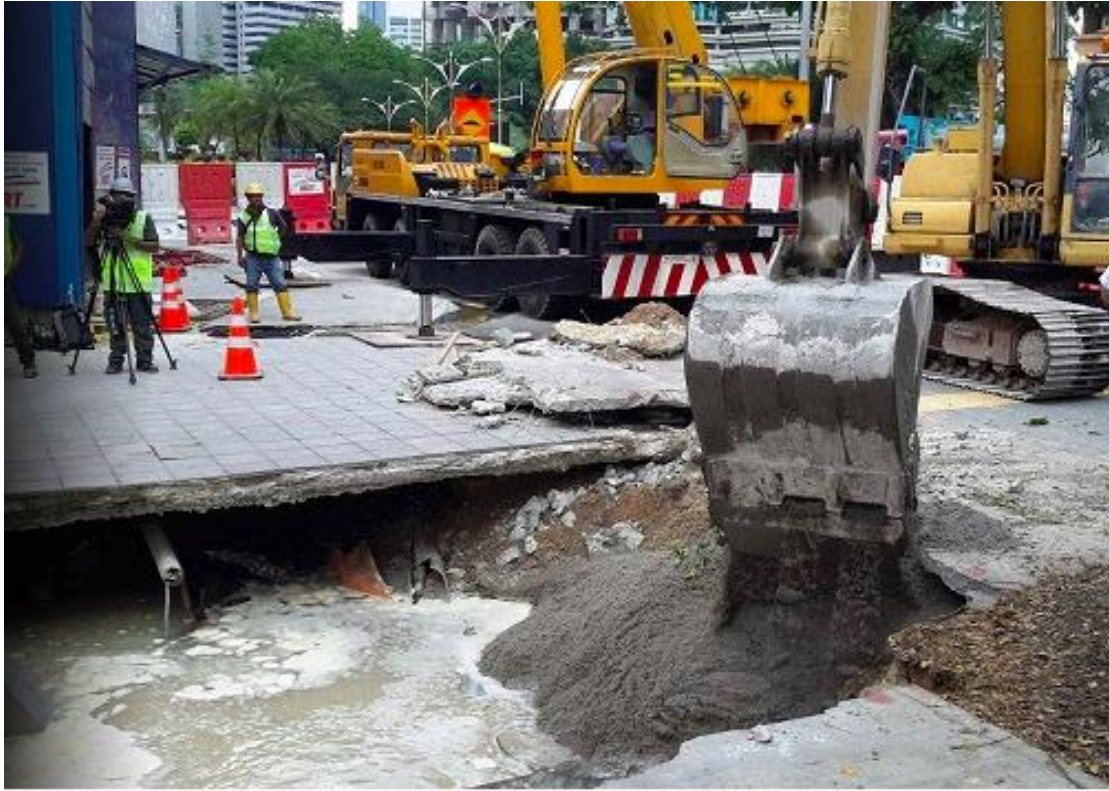
Figure 7: Sinkholes at Jalan Bukit Bintang 6m from MRT tunnelling construction (Courtesy: MRT Corp)
