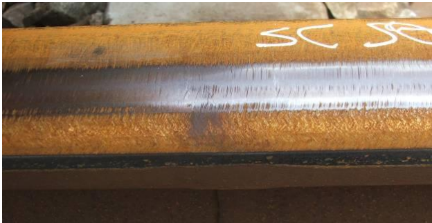
Fig. 8. Squat at flashbutt weld in SC rail which is otherwise squat free. Measured hardness 305-312HB in parent rail and 372HB in weld. High rail in arc of 872m radius curve [5].
