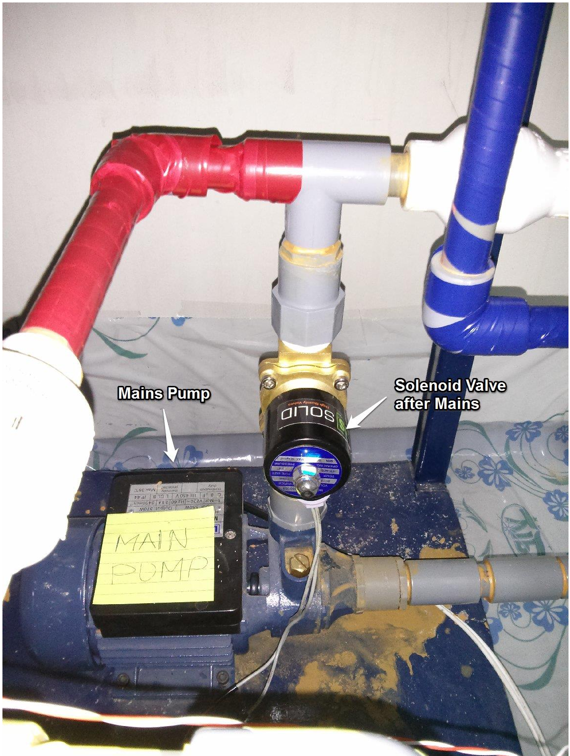
Figure A-4: Solenoid Valve places after the Mains
