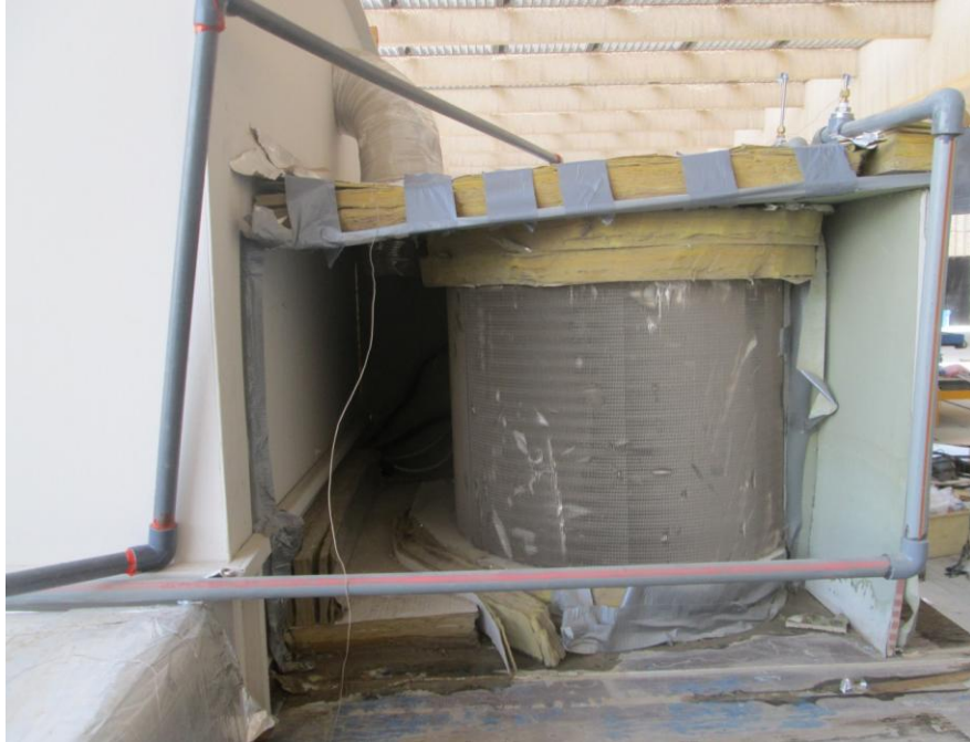
Figure A-6 Pre-cooler for option 'B' after installation.
