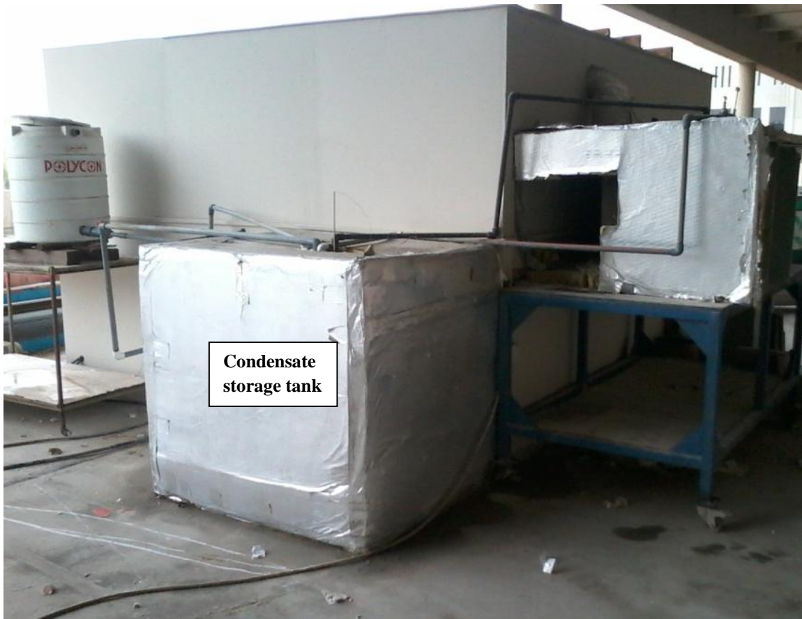
Figure A-12 Photograph of the experimental set-up outside the room showing the outdoor unit and condensate-storage tank.
