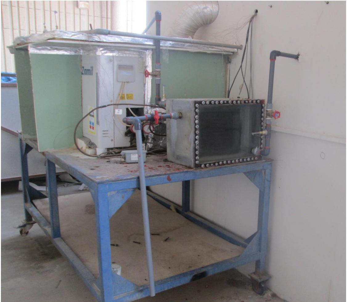
Figure A-10 Picture of the subcooler after installation.
