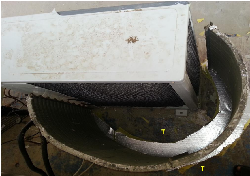
Figure A-5 Installation of pre-cooler for option 'B' behind the condenser.
