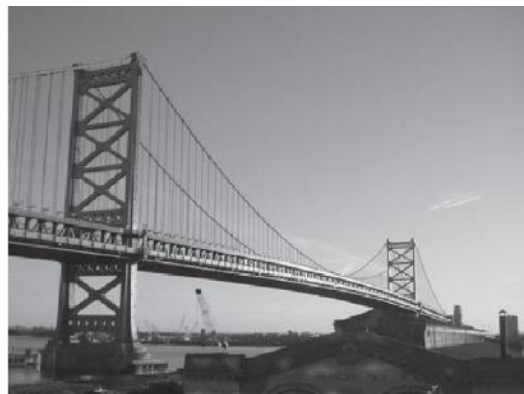
Fig. 6. Ben Franklin Bridge
