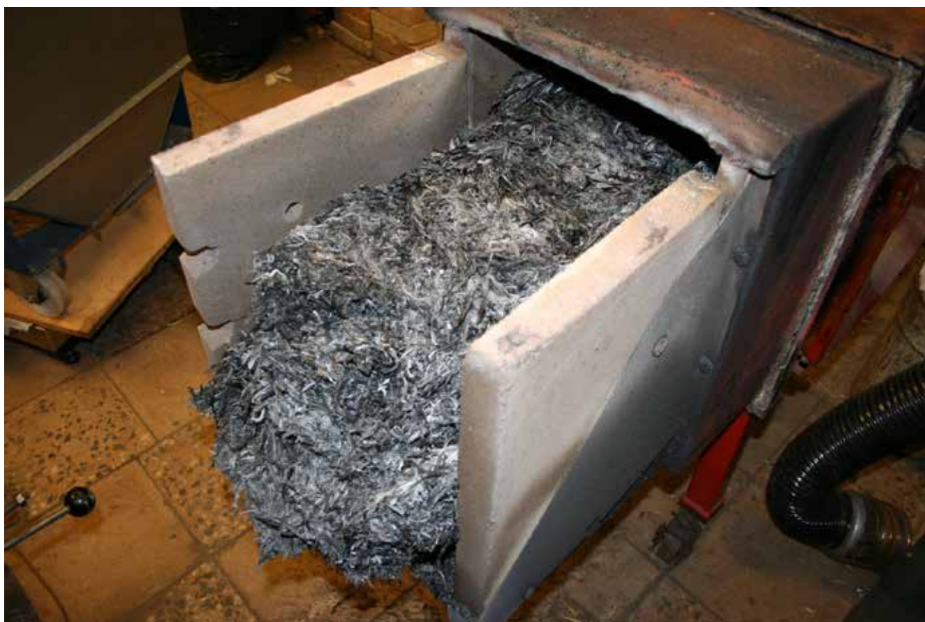
Figure 2. Reed ash in the grate of a stoker burner.
