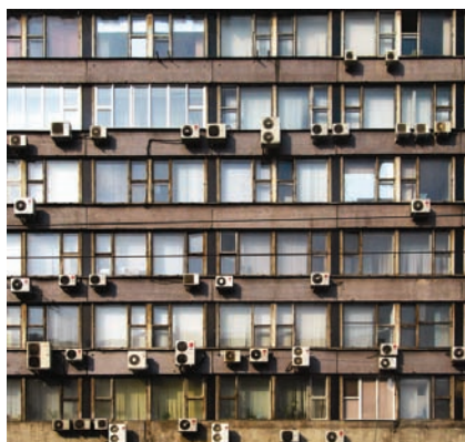
Figure 1. The facade of a multi-storey building from the 1960-80 period
