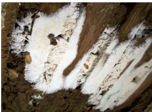
Photo 6 – The rapid expansion of mycelium of Peziza domiciliana Cooke in the floor, historical house, Stefan cel Mare Street, 75, Targu Neamt
