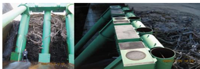
Figure 2. Sediment and driftwood trapped by the open check dam (beam type) in the Hachimandani River.
