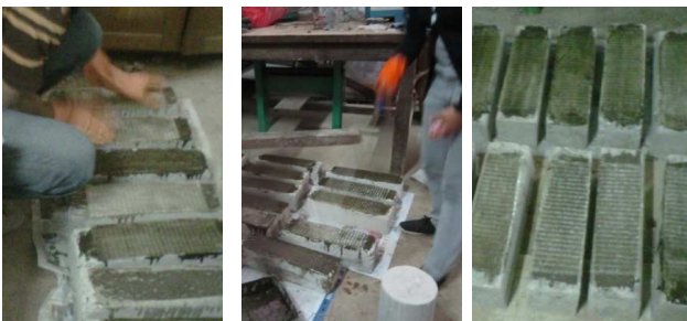
Fig. 3. Installation of GFRP Sheet on the beam
