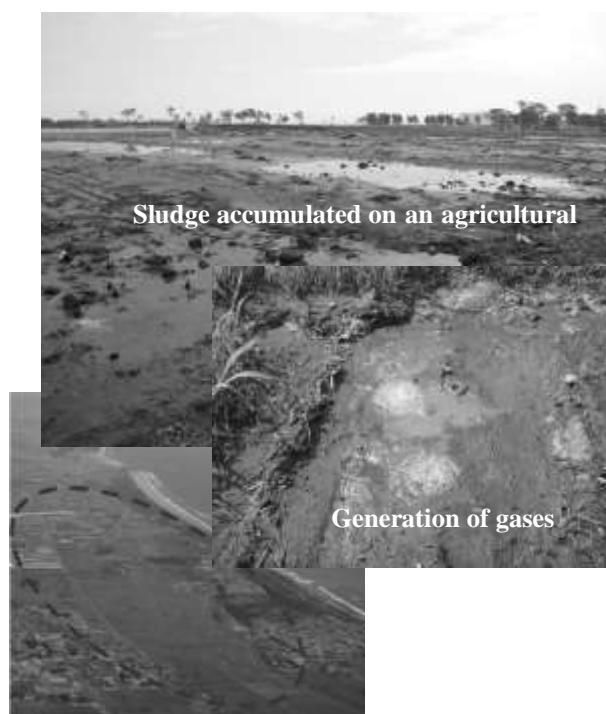
Fig. 1 Accumulated sludge after the Great East Japan Earthquake
