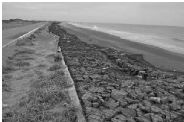
Fig. 22 Gabions placed along the coastline.
