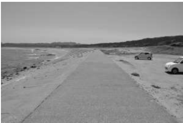
Fig. 7 A wide concrete walkway.
