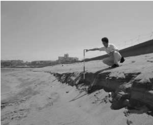
Fig. 2 Measuring of scarp height.
