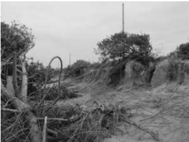
Fig. 19 Damage to the landward slope of a sand dune by the tsunami overflow.
