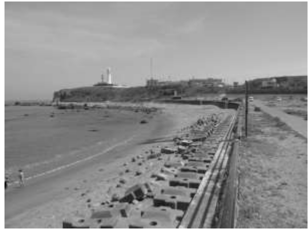
Fig. 4 Concrete blocks placed along the coastline to prevent wave overtopping.
