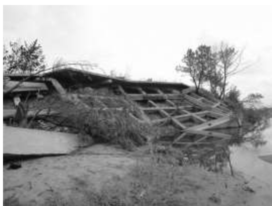
Fig. 1 Damaged coastal dyke in Tohoku after the 2011 Tohoku Earthquake and Tsunami
