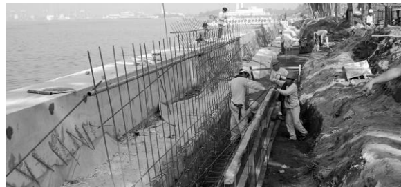
Fig. 8 Rehabilitation of RB seawall after T.Pedring
