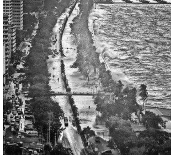
Fig. 7 (left) The seawall overtopped and Roxas Blvd flooded during TS Gener.
