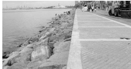
Fig. 3 RB seawall before Typhoon Pedring occurrence
