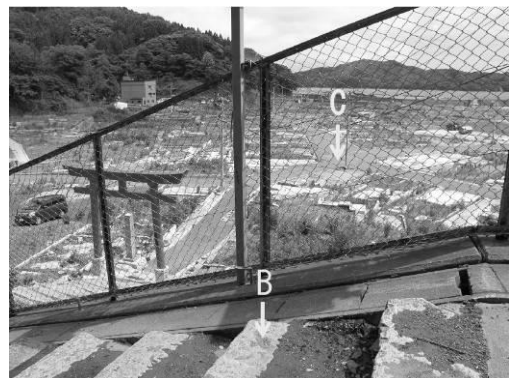
Fig. 5 The tsunami reached the second step below the top of the stairway (arrow B).
