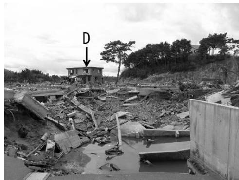
Fig. 21 Destroyed coastal dike.
