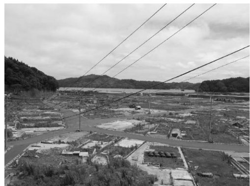
Fig. 6 Seawall along Ootsuchi Bay and damaged area.
