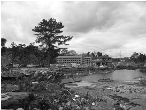
Fig. 19 Tsunami damage immediately inland of coastal dike.
