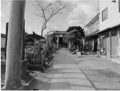
Fig. 24 Destroyed house next to Suwa Shrine.
