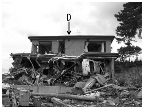
Fig. 22 Destroyed house and debris inside it.
