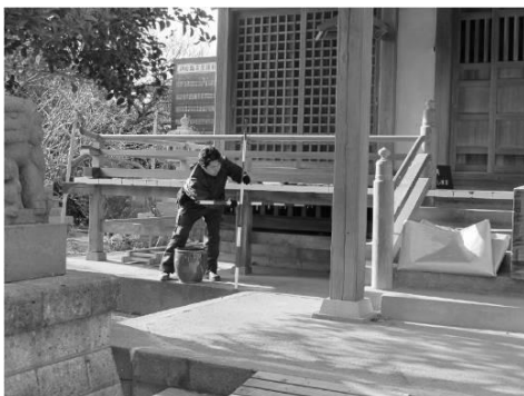
Fig. 26 Clearance under floor of the shrine.
