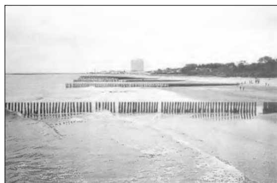
Fig. 1 Permeable groin Baltic Sea, Jerman (Raudkivi, 1996)
