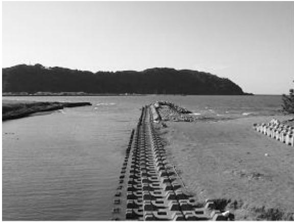
Fig. 15 Impermeable jetty constructed.
