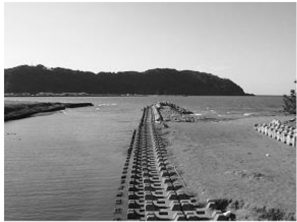
Fig. 15 Impermeable jetty constructed.
