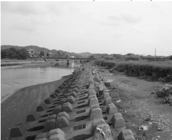
Fig. 7 Concrete blocks inclined toward the channel (October 13, 2011).
