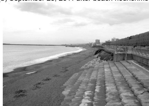
Fig. 2 Foreshore changes on Chigasaki coast between August 29, 2005 and September 25, 2011 before and after beach nourishment, respectively
