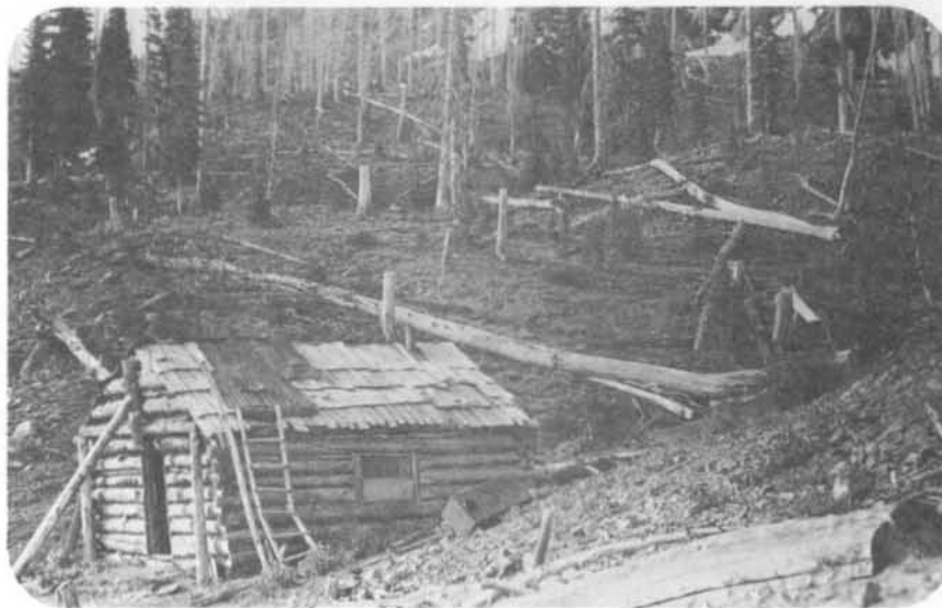
The old Potosi cabin near Windy Gap in the Greenhorn Mountains, one of the oldest mines in the Greenhorns. Nearby mines included the Ben Harrison, Morris, and the Bi-metallic. Picture taken in July, 1917. Notice snow in background and snow-broken shakes along eaves. Cabin is at an elevation of 7000 feet above sea level.
