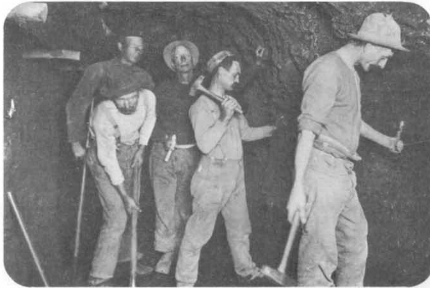
Miners and muckers at the Bonanza mine, 1894. Note use of wax candles and "single jacks" -- 4-pound hammers used with hand-held drill steel. Discovered in 1877 by Jack Haggard, the mine was sold for $350 in 1879 to the Bonanza Mining Co. In 1892 it was purchased by the Geiser Brothers, who took out about $400,000 before selling it to the Pittsburg Mining Co. for $500,000. The mine was eventually worked to a depth of 1200 feet with a production estimated at approximately 1-3/4 million dollars at the old $20.67 per ounce price of gold. Geiser, a town located at the mine, boasted a post office between July 15, 1898 and June 15, 1909.
