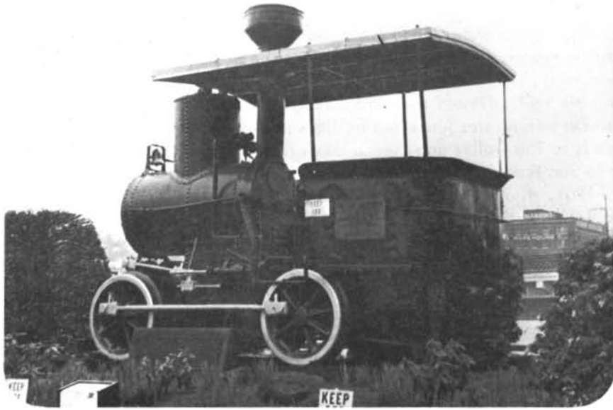
This small engine, on display at the Union Station in Portland, was named "The Pony." It was built in San Francisco, then shipped to the Cascades in 1862 to help speed up the traffic over the portage. The rails were made of wood covered with strap iron. This was Oregon's first railroad. (Oregon Historical Society photograph)
