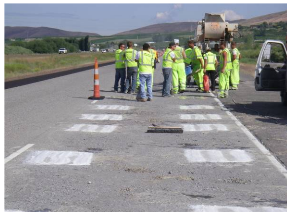
Figure 13. Finished installation prior to diamond grinding to remove faulting.
