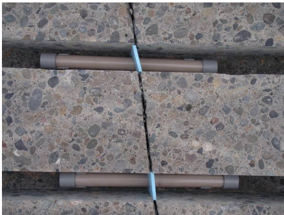
Figure 6. Close-up of dowels in slots.
