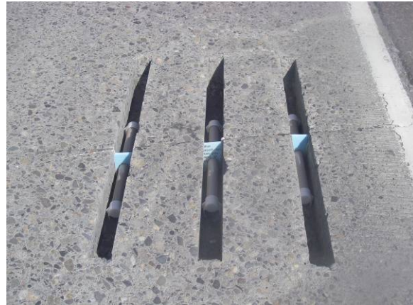
Figure 9. Dowels in slots.
