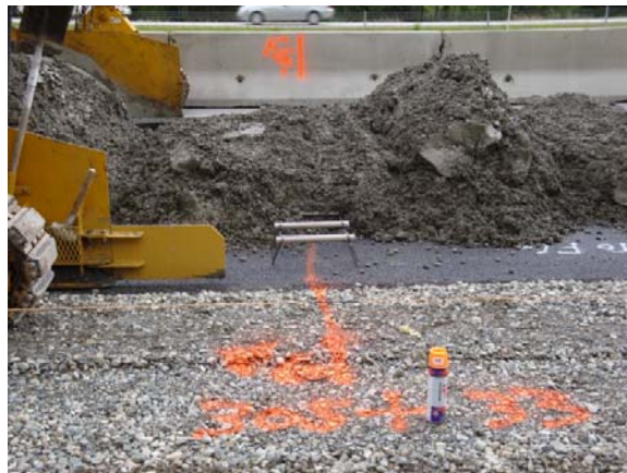
Figure 3. GFRP dowels used in new construction on I-5.
