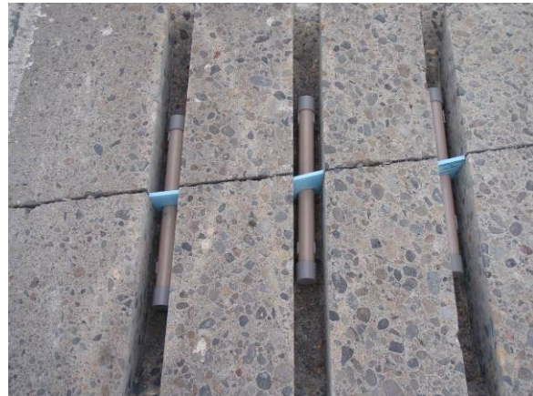
Figure 5. GFRP dowels placed in slots.
