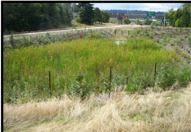
I-405 Bellvue Combined Stormwater Treatment Wetland/Detention Pond
