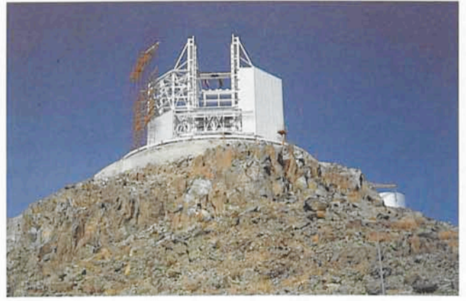
Figure 3: The rotating building under construction in April 1988.
