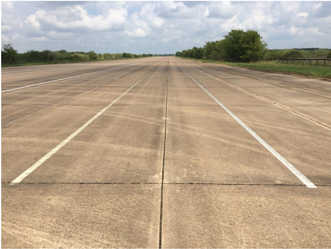
Figure 5. Layout of Closed Course Pavement Markings for Repeatability Analysis
