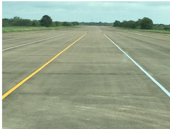
Figure 4. Pavement Marking Layout for Closed Course Correlation Analysis
