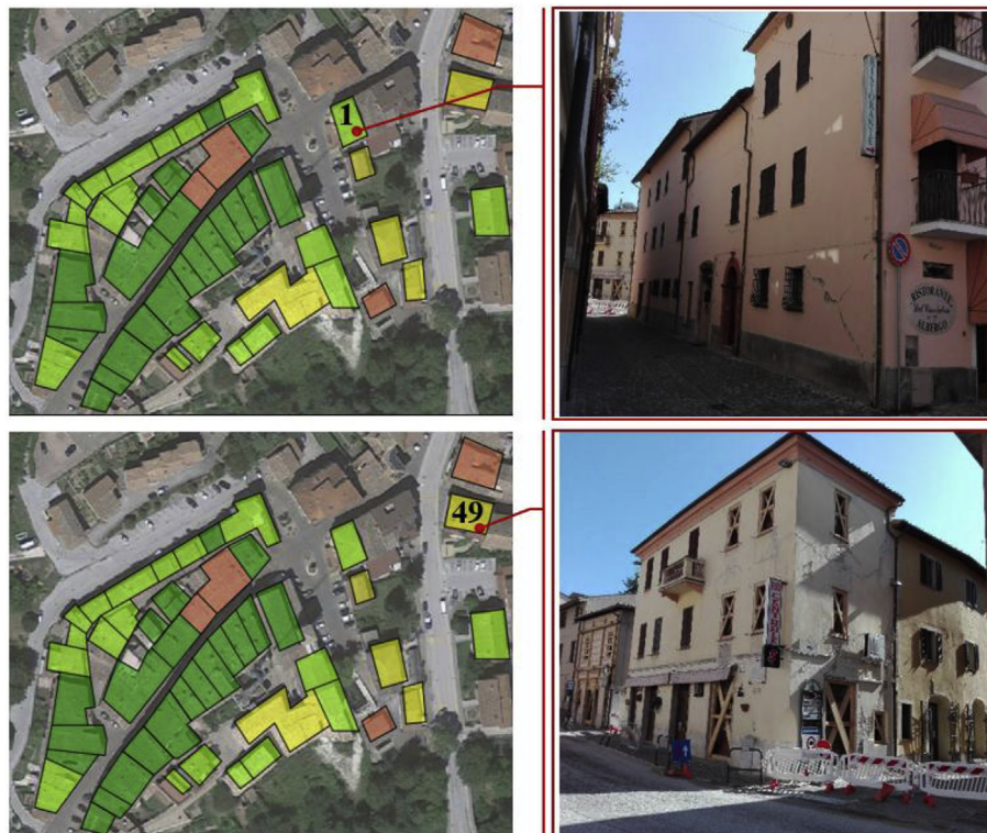
Fig. 13. Correlation among analysed damage scenario and site-inspection.
