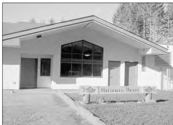
FMCC's Holloway House induction unit (2000) Corrections Branch Archives
