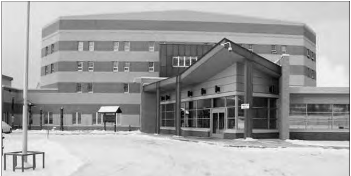
Prince George Regional Correctional Centre (2003) Corrections Branch Archives
