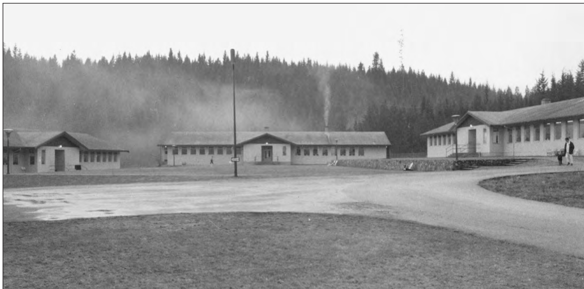
Living units at Alouette River (date: unknown) Corrections Branch Archives
