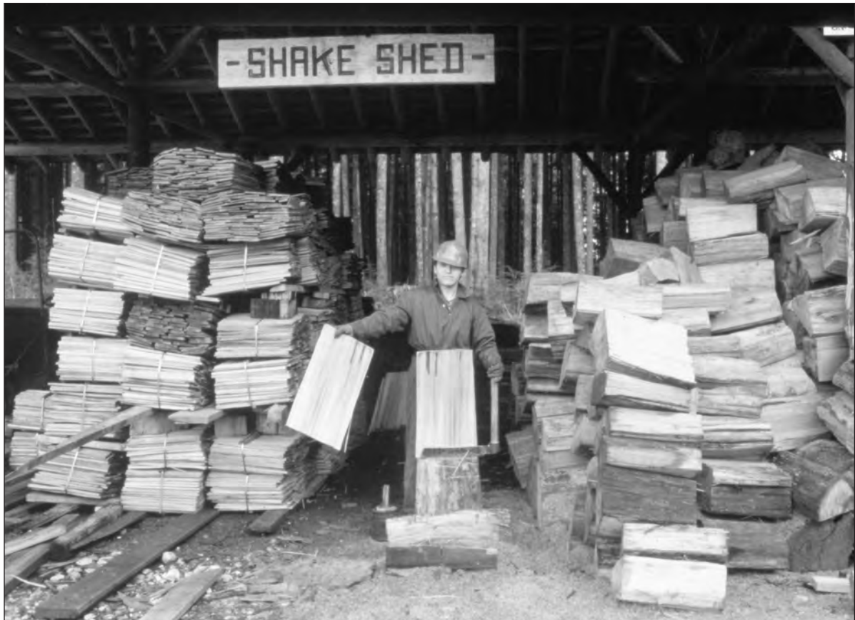
Cedar shake program at Stave Lake (1985) Corrections Branch Archives
