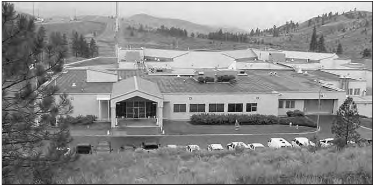
Kamloops Regional Correctional Centre (2002) Corrections Branch Archives
