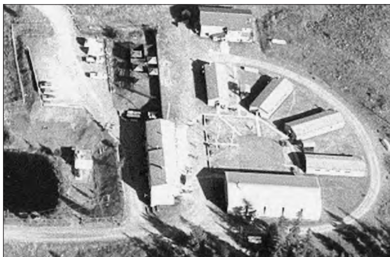
Overview of Bear Creek Correctional Centre (2002) Corrections Branch Archives
