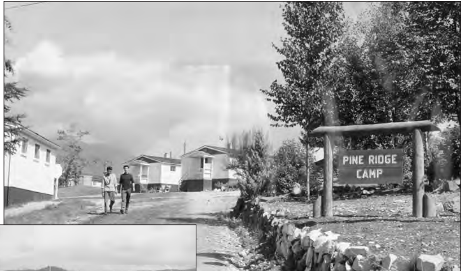
Pine Ridge (1964) Clockwise from right: Entrance to camp; Administration building (date: unknown); Fremwood project; Camp overview Corrections Branch Archives
