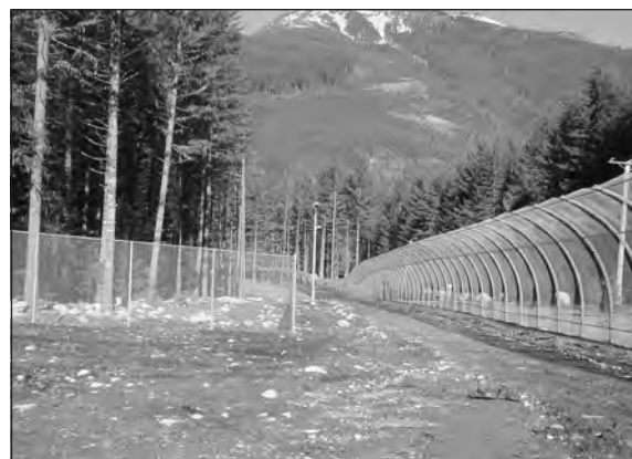
Perimeter fencing surrounding FMCC (2000) Corrections Branch Archives
