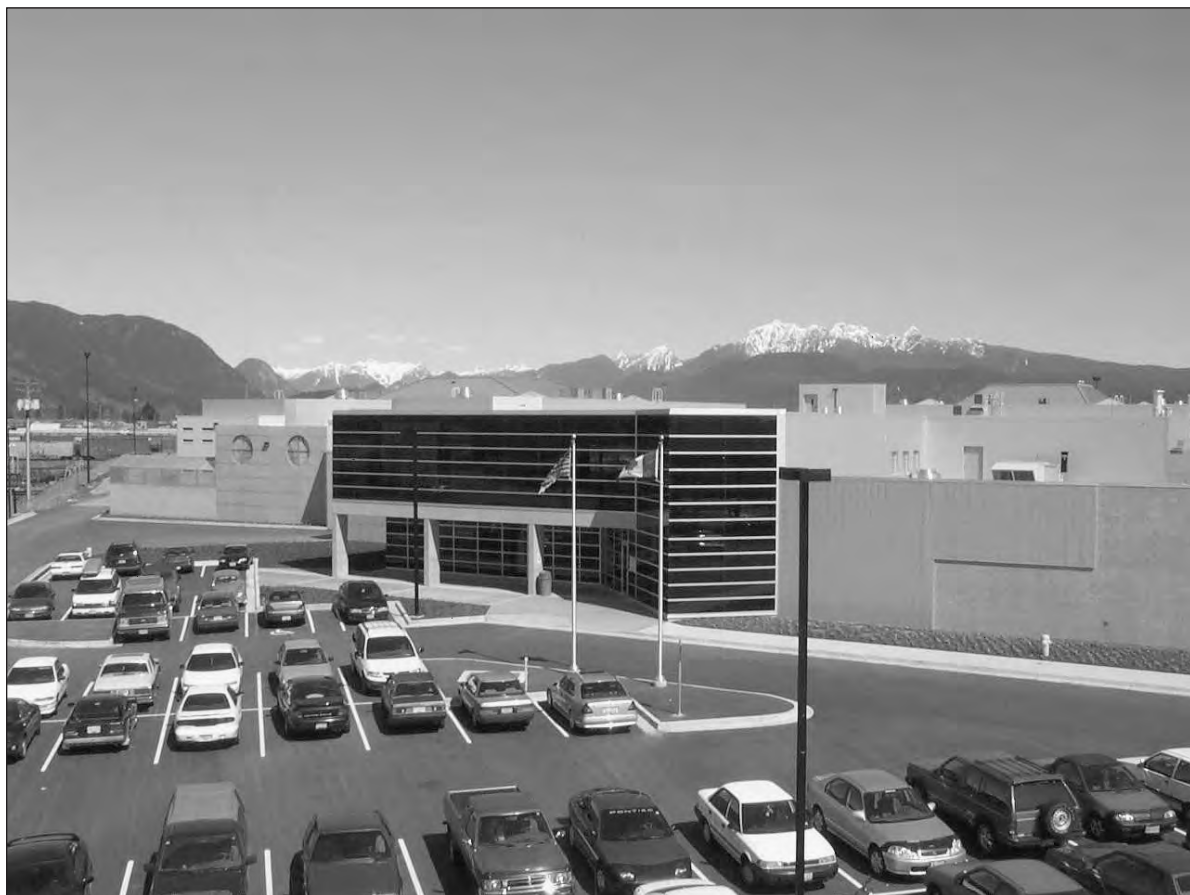
Entrance to North Fraser Pretrial Centre (2002) Corrections Branch Archives
